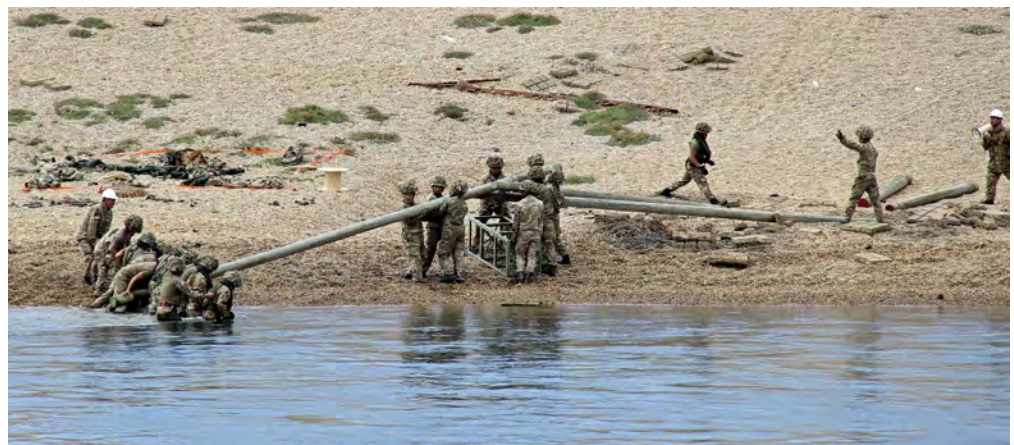
Assembling a tripod to provide an aerial ropeway to transport soldiers and equipment across the gap
