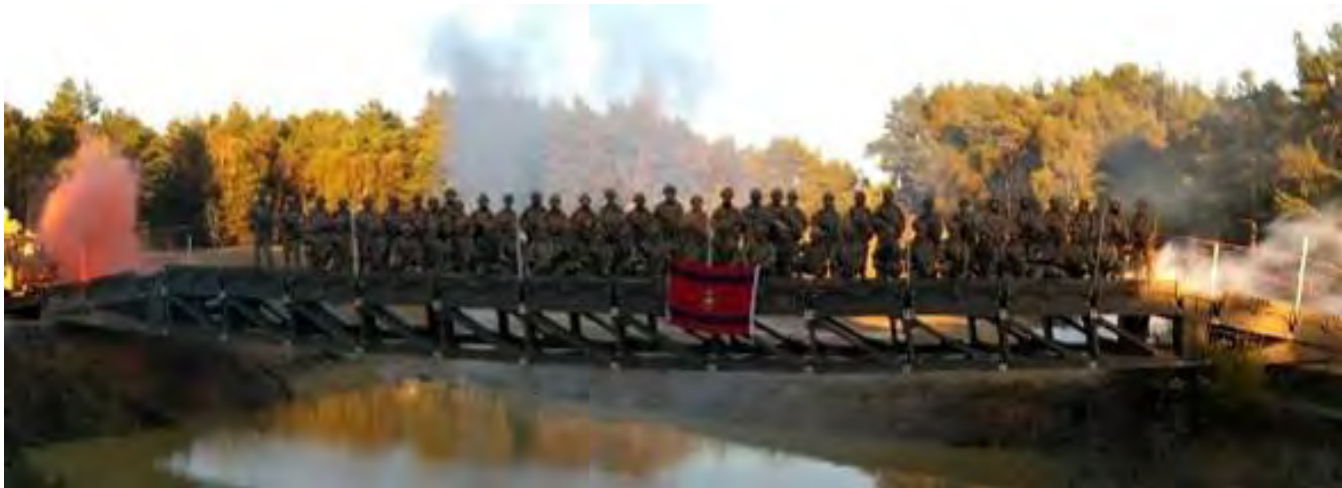
A full Squadron effort for the 12-bay double storey medium girder bridge
