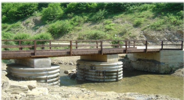
The Devic Bridge
