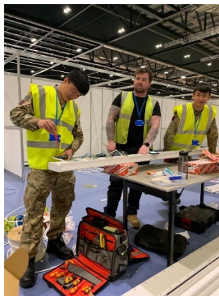
Civilian and military tradesmen working together while LCpl Mahesh installs MDF board to support a cubical
