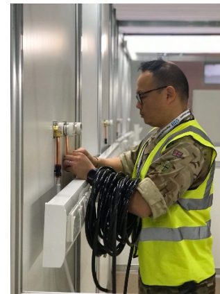
LCpl Nirpesh (left) preparing trunking for ICU cubicles, while Cpl Ganga installs a medical air supply connection
