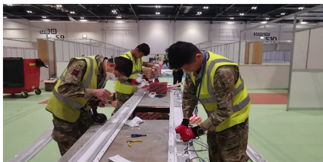
Military and Civilian Electricians preparing trunkings for ICU cubicles
