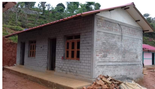
A typical brick house with sandwich roof
