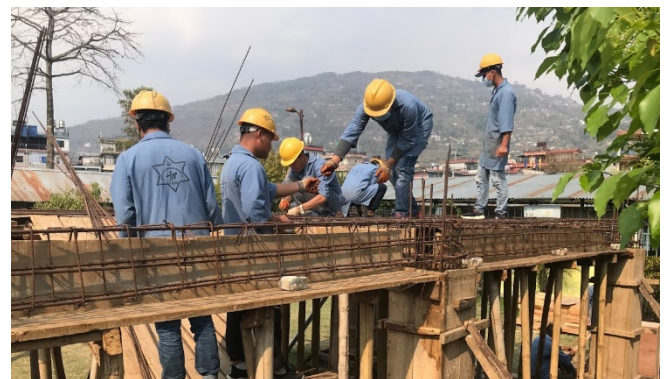
Employment Training: Shuttering and Steel fixing
