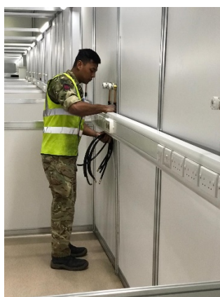
LCpl Nirpesh (left) preparing trunking for ICU cubicles, while Cpl Ganga installs a medical air supply connection
