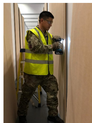
Civilian and military tradesmen working together while LCpl Mahesh installs MDF board to support a cubical
