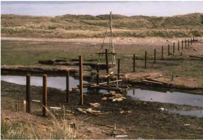
The improvised pile driver, dreamed up by the Gurkhas
