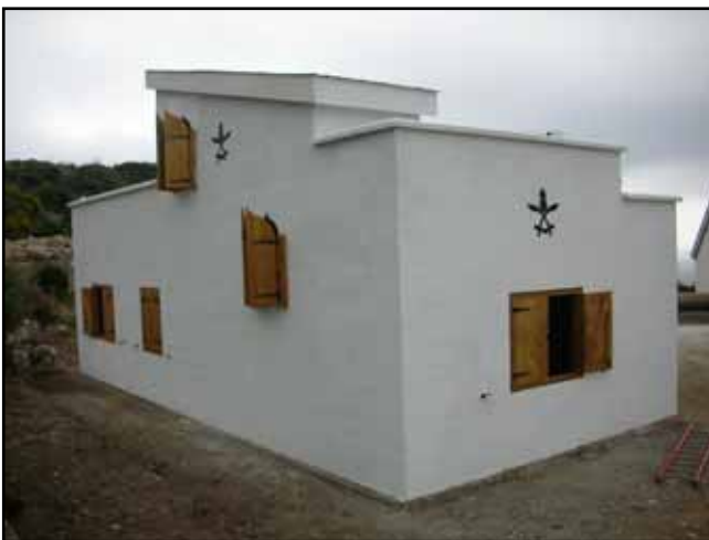
The completed FIBUA house on Ex 28 th SHOT
