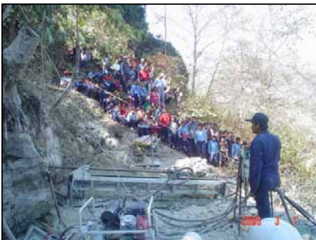
Horizontal Drilling at Mulabari village in Syangja district
