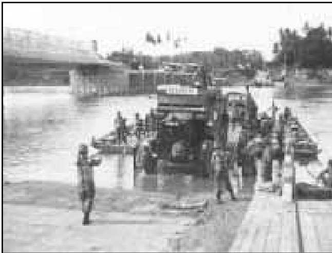
Temerloh Ferry, Malaya operated by Gurkha Engineers c1950's (Photo: Unknown) – Taken from RE Museum Homepage
