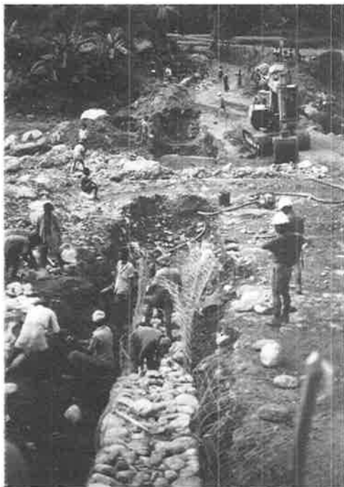
'C' Troop constructing the downstream gabion basket wall.
