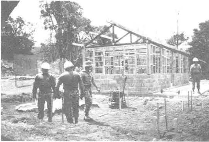
Construction of NCO accomodation.
