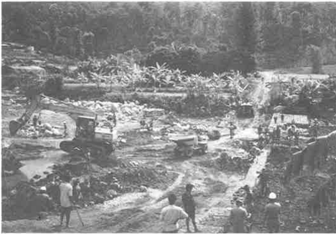
The construction site - Day 7.
